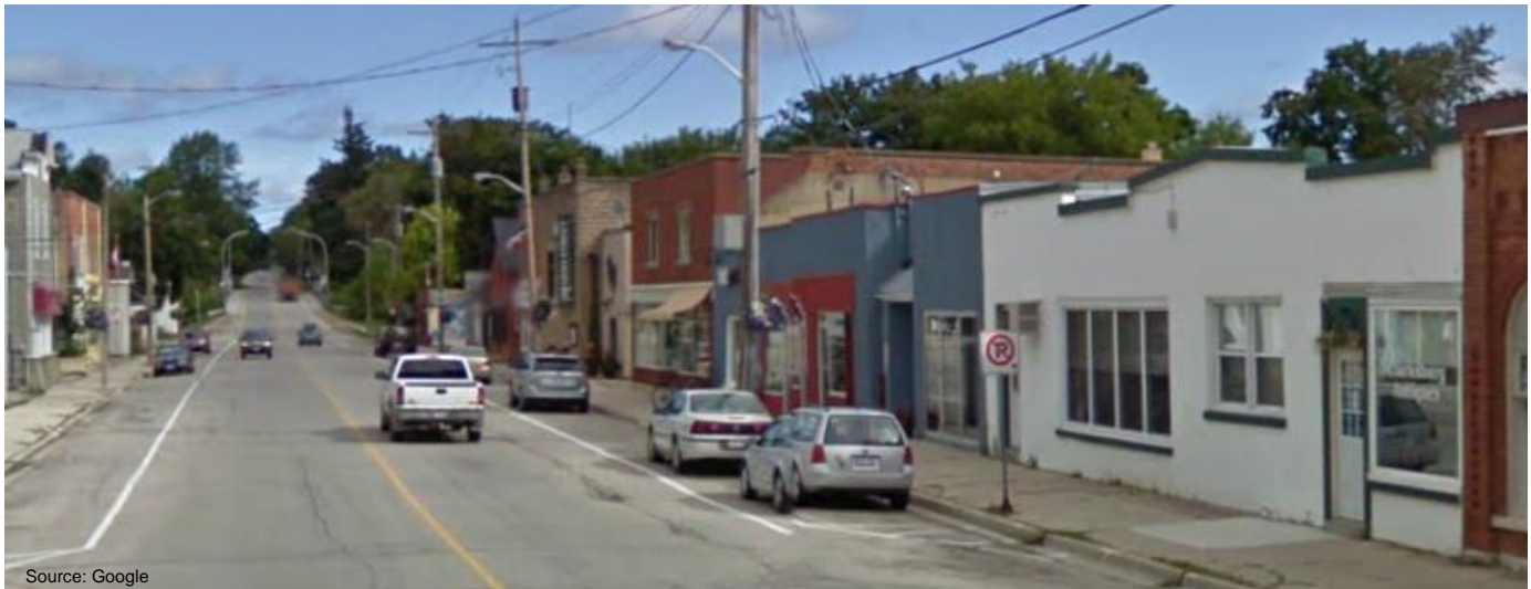
Clarksburg Commercial Core, Marsh Street
